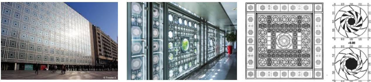
Figure (9): L’arab du monde institute adaptive façade Source: https://www.archdaily.com/ , Accessed June, 2020
